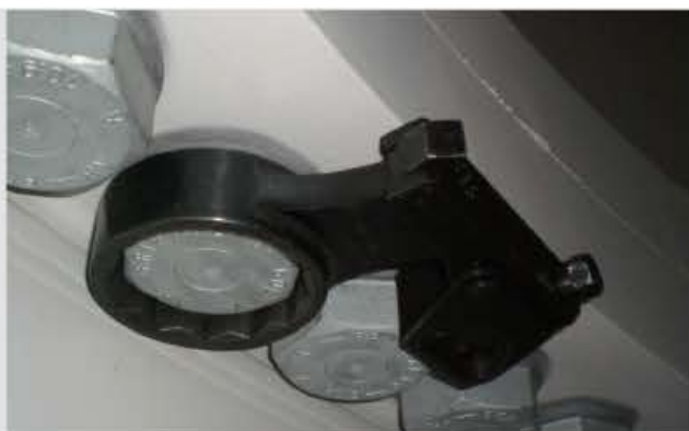
alkitronic® backup wrench in use on the bolt circle in a wind power plant.
